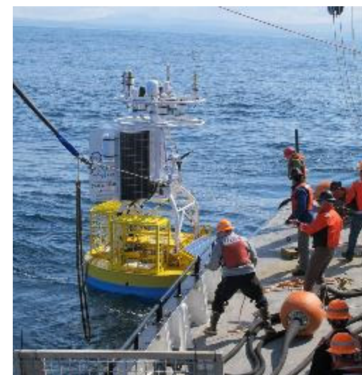
Endurance surface mooring deployment, July 2015.
