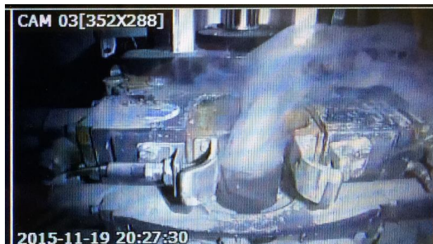
Figure 6. Schematic of borehole plug in M0072B. Screenshot of top of M0072B while drilling, before borehole plug was installed.
